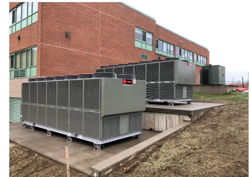
Middle School Chillers
